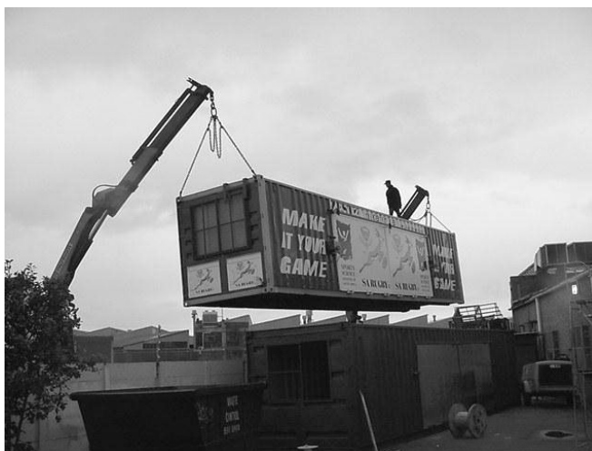
Figure 1. A Mobile Gym Being Hoisted onto a Truck at the Factory Before Being Transported to a Club
